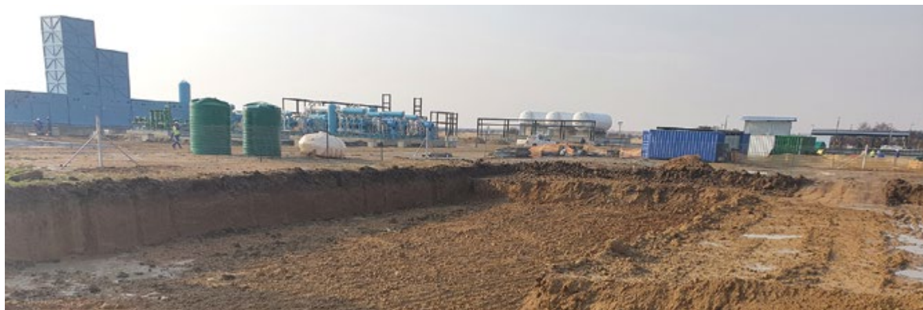
Construction of water circulation reservoir.
