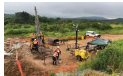
Drilling taking place at New Luika gold project.
