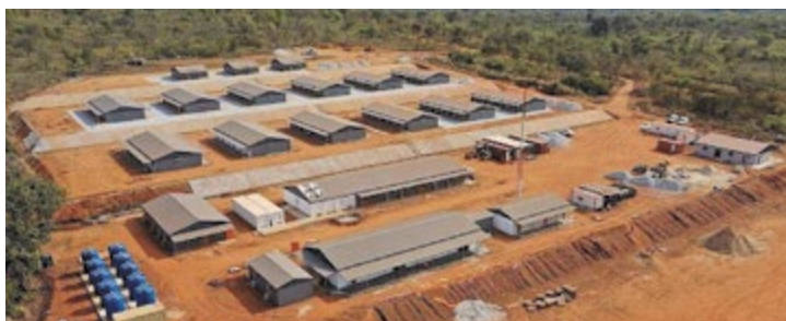
A 156-person accommodation camp being built at the Séguéla gold project.
