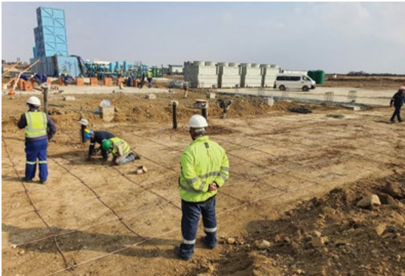
Above: Laying foundations for large compressors.
